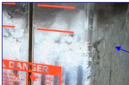
Gelled Electrolyte VRLA Battery Construction
